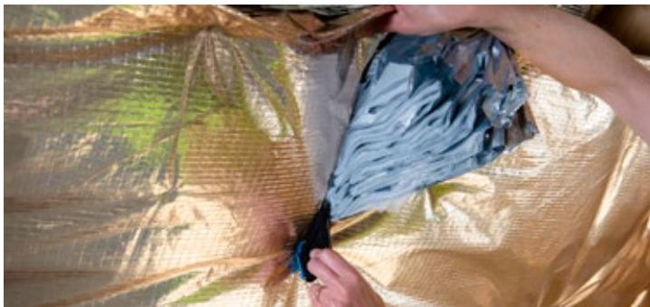
**Eolis HC** can easily be cut using an **ACTIS** cutter or a sharp knife. Align a timber batten where the product is fixed onto rafters and cut along pressing the timber batten firmly onto the product. Alternatively an electrical circular shear tool can be used.
