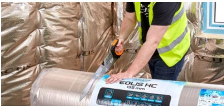
If the product is required to be cut lengthwise, it is recommended that this is carried out whilst the product is still in its packaging using an insulation saw.
