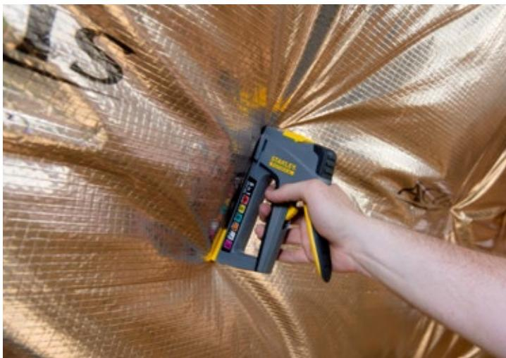
Install **Eolis HC** across the face of timbers fixing in a continuous layer. Maintain insulation thickness by making sure that the product is not pulled too taut and that the insulation fills the space required to accommodate product thickness. Staple to timbers every 250mm, using min. 14mm galvanised staples.
