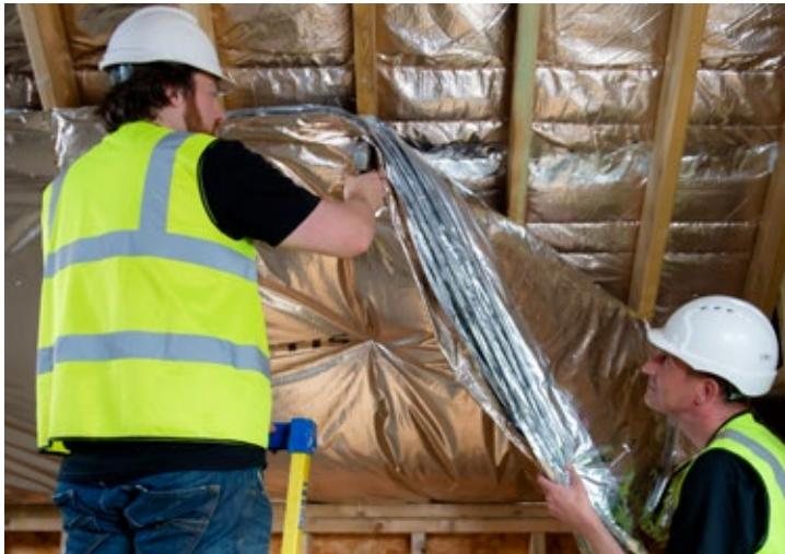
Remove the packaging e.g. by using an **ACTIS** cutter. Use **Eolis HC** with the reinforced (grid pattern) copper-coloured film facing the inside (warm side) of the building.
