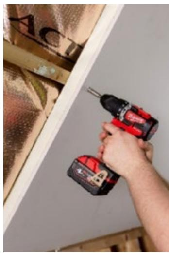
Butt-join **Eolis HC** with the next layer of the product. Peel back the paper from the built-in self-adhesive tape and bring the entire overlap in contact with the lower layer sealing securely. Vertical joints are to be sealed with **ACTIS** tape which is recommended for the product.
